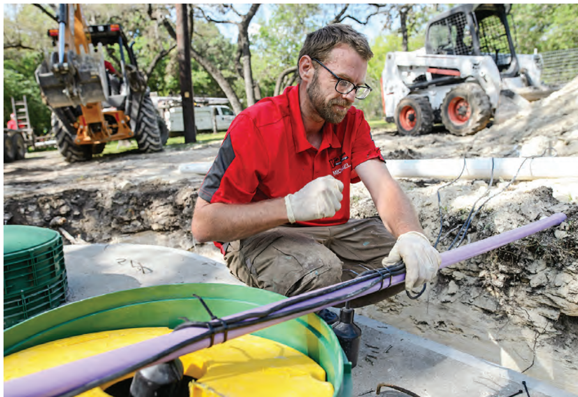
⚡ Michael Foley works on electronic components while installing a residential septic system. Van Delden Wastewater Systems installs about 80 systems annually from Clearstream Wastewater Systems.
