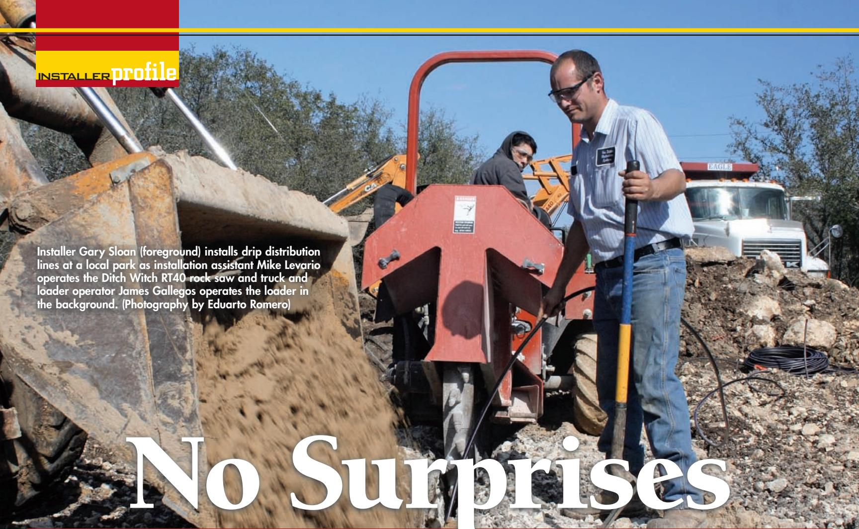
Installer Gary Sloan (foreground) installs drip distribution lines at a local park as installation assistant Mike Levario operates the Ditch Witch RT40 rock saw and truck and loader operator James Gallegos operates the loader in the background. (Photography by Eduardo Romero)
